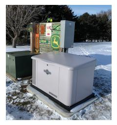
a house. 1340301 This type of generator is permanent but not considered "standby" because of the manual switch, and it should not be located near a home. (Consult a professional electrician when installing or maintaining a permanent generator.)
